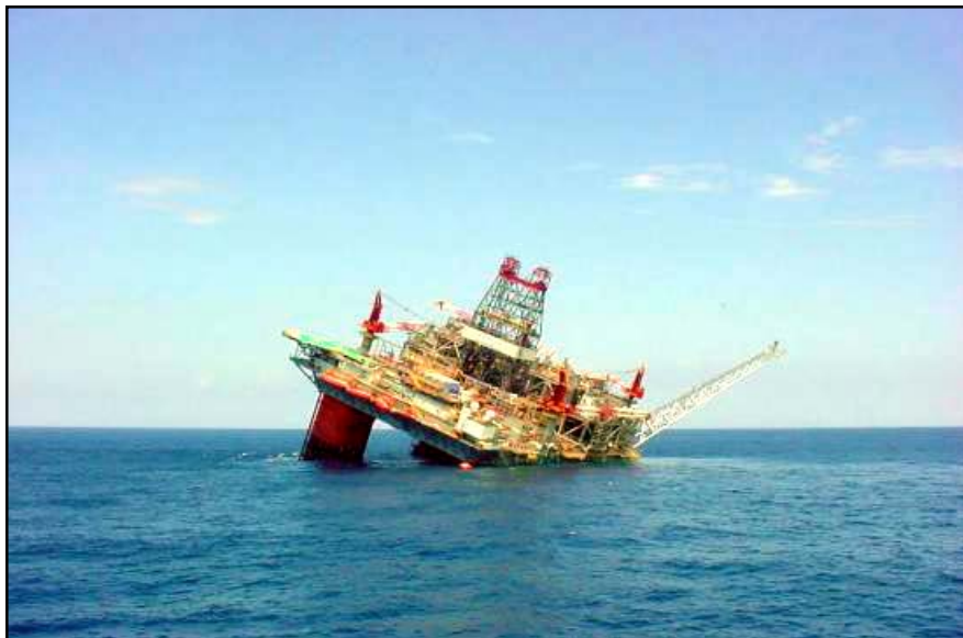
The Thunder Horse oil rig following a riser break in 2003. Photo courtesy of NOAA/Department of Commerce.
